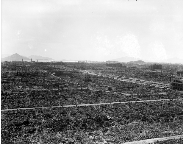
(a) Total Destruction Near the Epicenter
